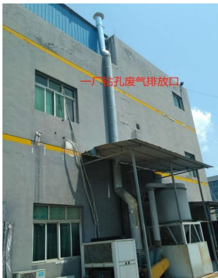
钻孔工序+15m 排气筒
